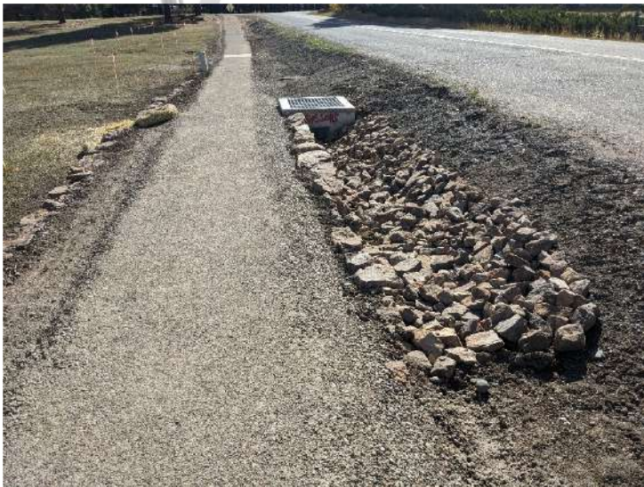
Figure 3 Outlet Structure & Drainage Improvements on the Northlake Avenue Pedestrian Trail, a 4' wide gravel trail.
